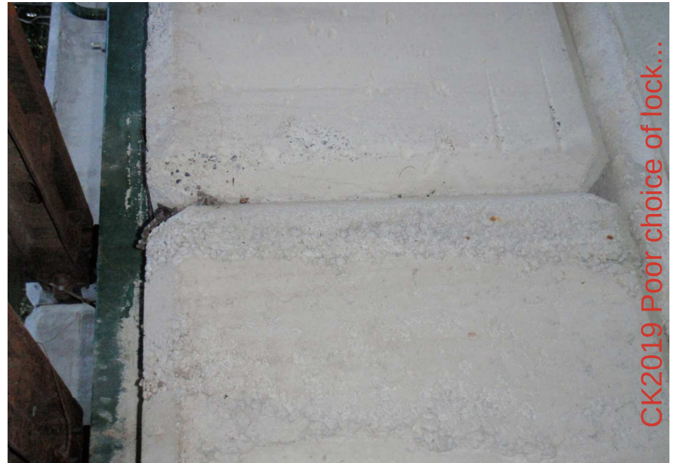
CK2019 Poor choice of lock block
